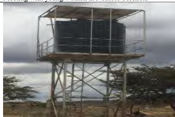
Ilkiroti community = borehole fitted with solar pump
