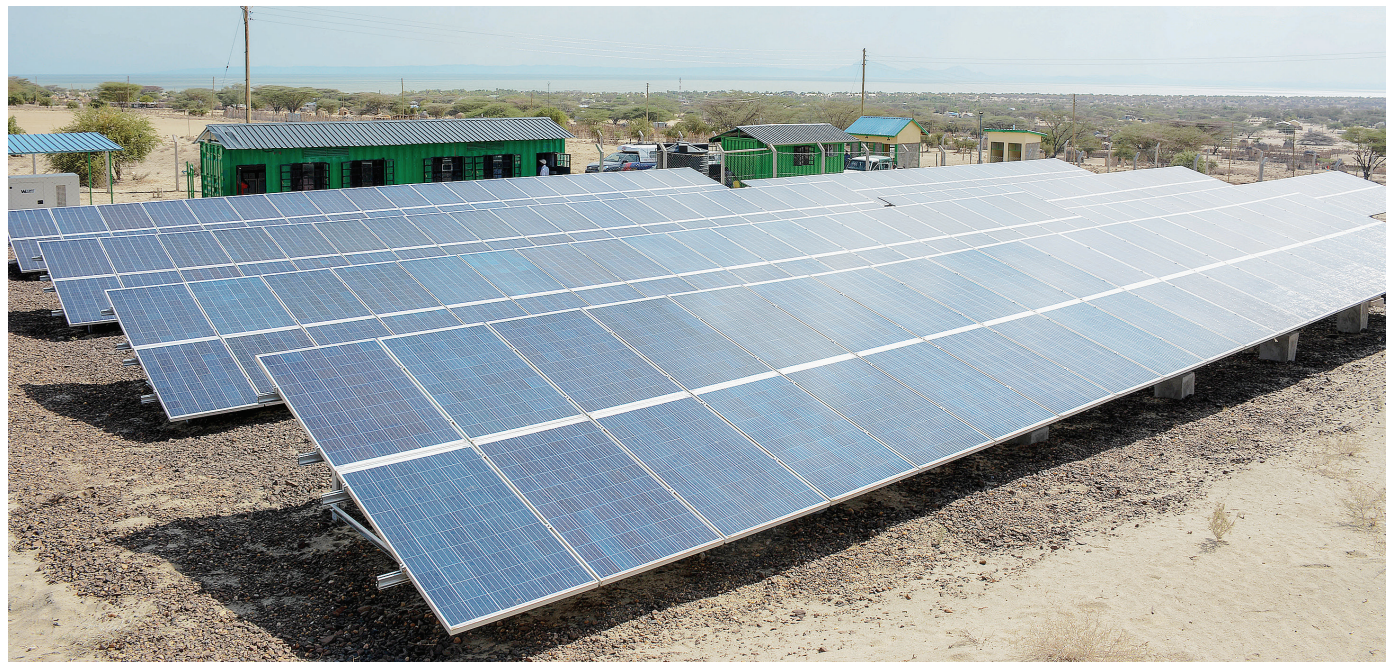
Eliye springs solar mini grid project in Turkana county.
