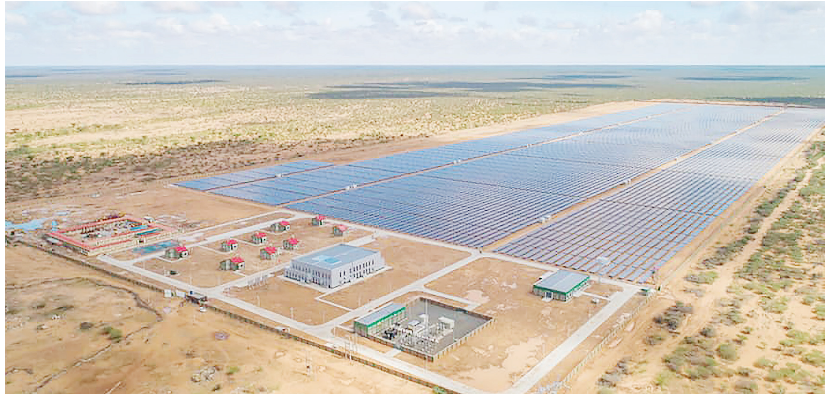
Aerial view of the 50MW Garissa Solar Project.
